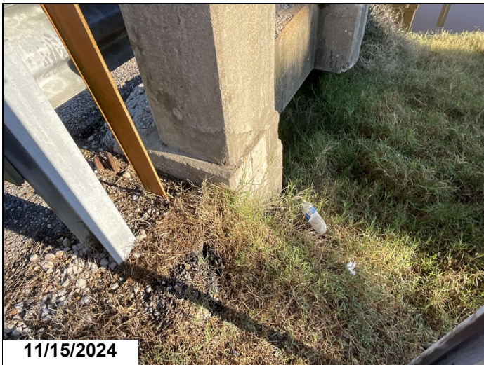
Bent 1 right wing is missing from past damage 11-15-2024
