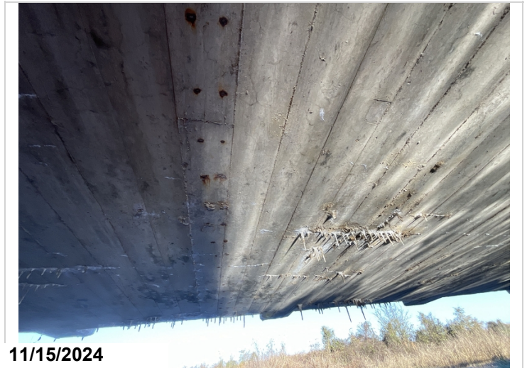
Span 1 left cracking with efflorescence 11-15-2024
