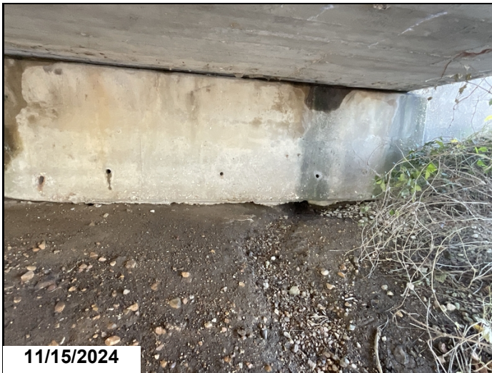
Bent 1 left end erosion 11-15-2024
