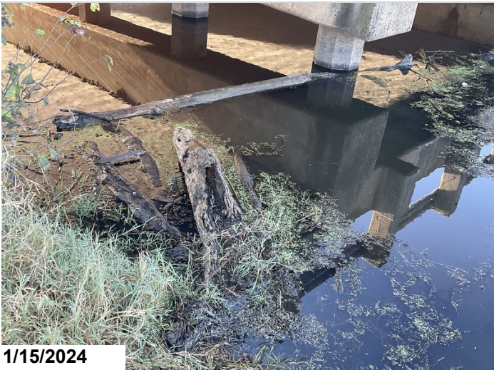
Drift lodged against bent 2 11-15-2024
