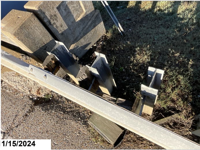
Bent 4 (East end) on left approach rail 3 wood spacer blocks damaged. 11-15-2024
