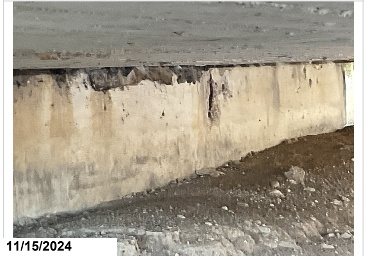
Bent 3 center line rebar 11-15-2024
